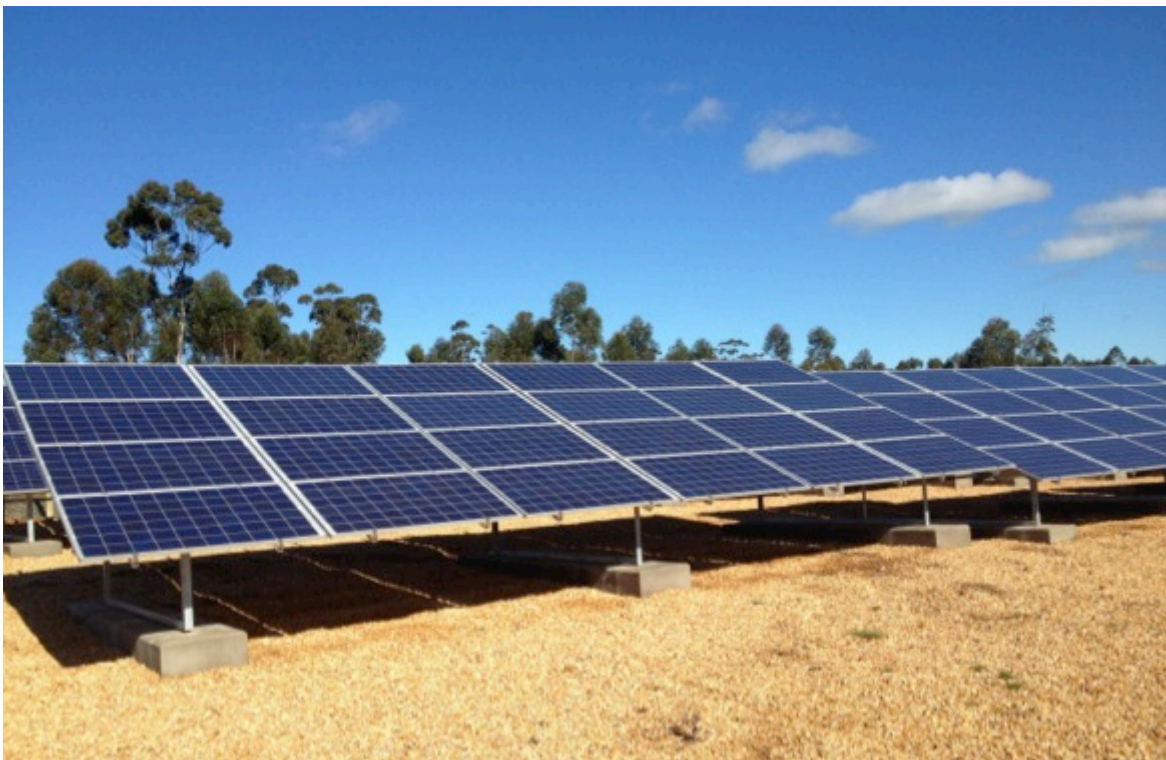
A 33 kW p PV municipal installation in Riversdale
