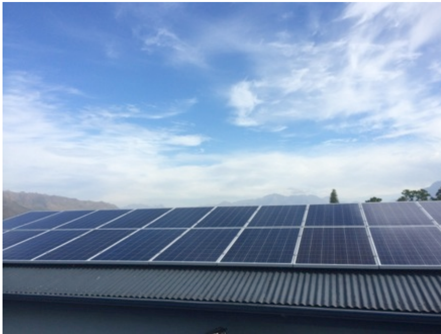
Figure 4.4: A 4.25 kW p PV installation at private residence, Paarl
