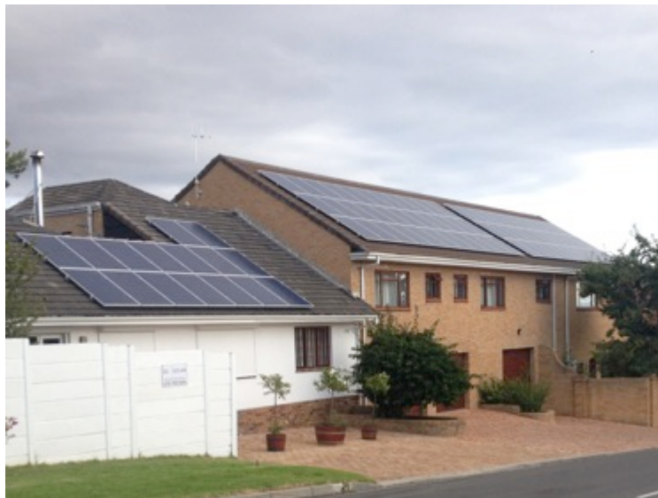
Figure 3.2: Rooftop PV installation at a guest house in Somerset West
