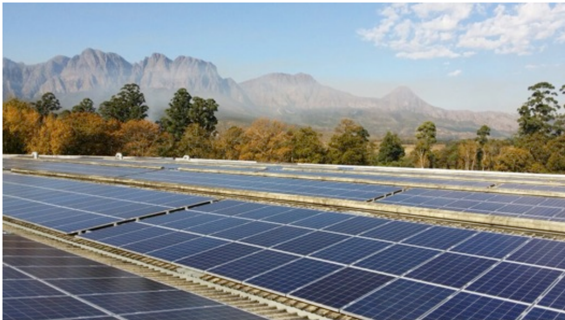
Figure 2.3: 500kW p PV installation at Lourensford Wine Estate, Somerset West
